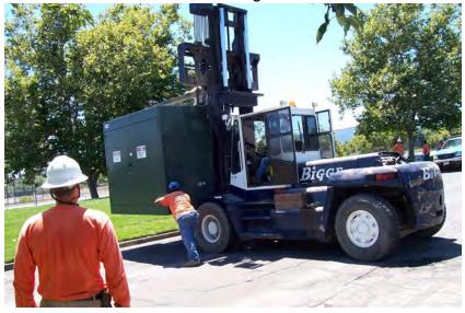
A new 10-ton transformer was installed under the watchful eye of workers.
